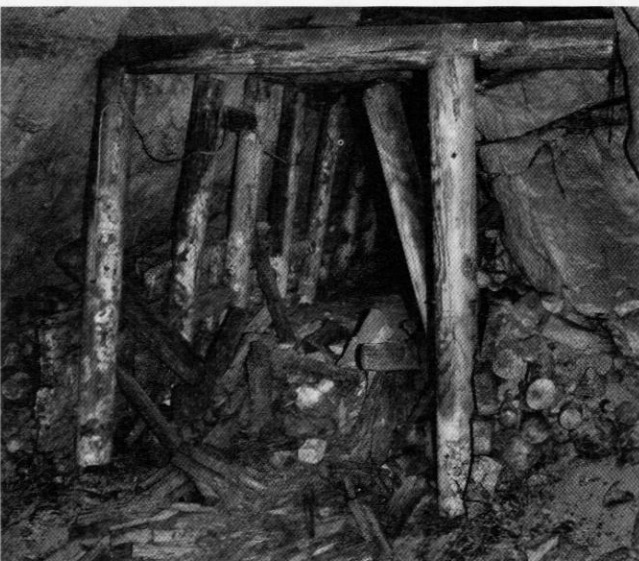
Unfinished tunnel leading to one of the ventilation shafts. Photo Tony Page
